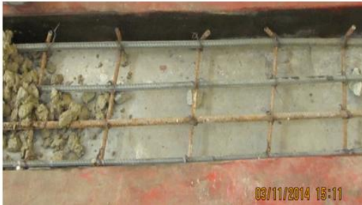
Fig. 4.3. Reinforcement in beam mould during casting.
